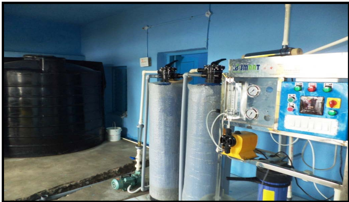
RO Water Plant Provided in Srinagar village
