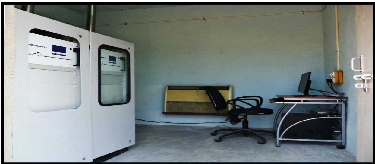
CAAQMS Station-3 installed at Mines area
